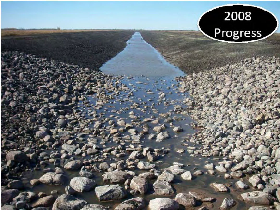
Figure 179. 2008 progress on restoration of Ditch 1
