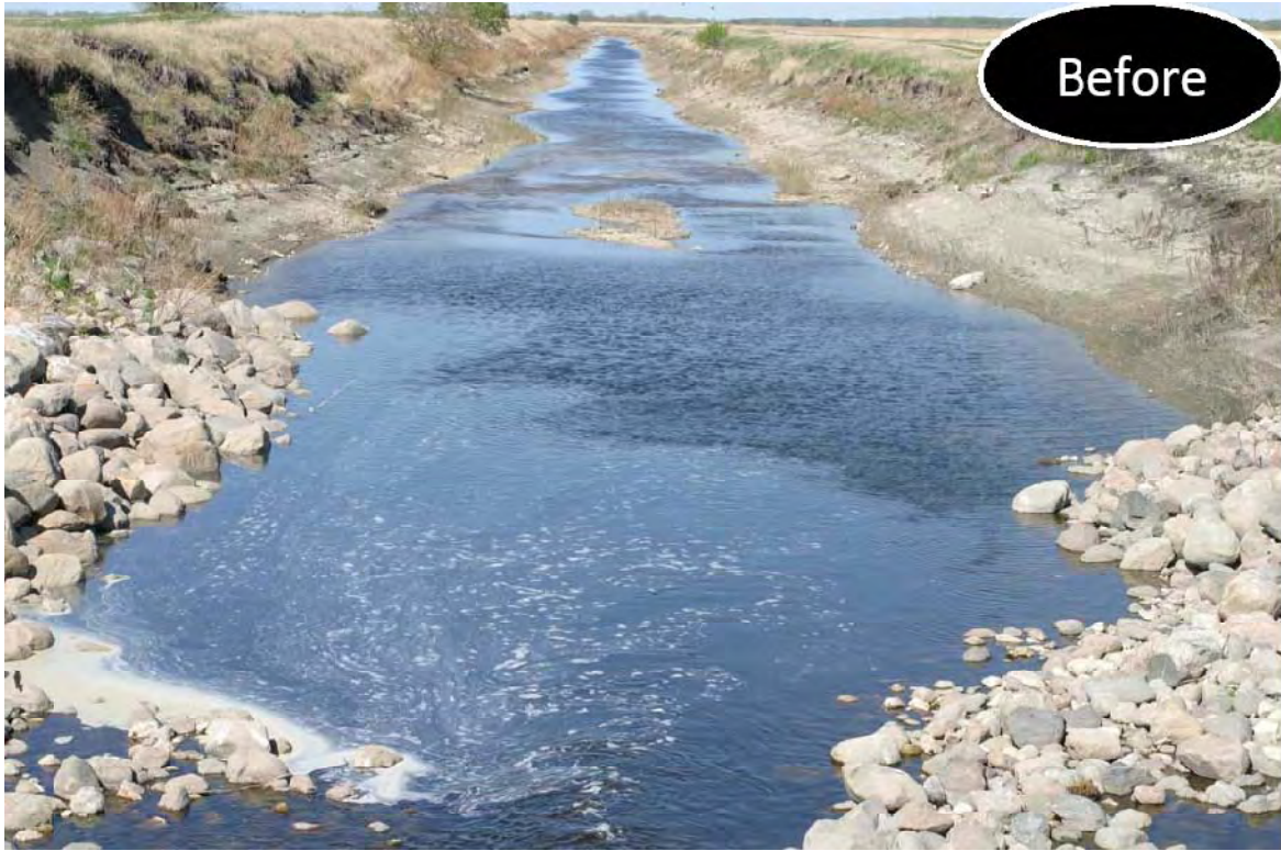
Figure 178. Stabilization of ditch 11 (before)
