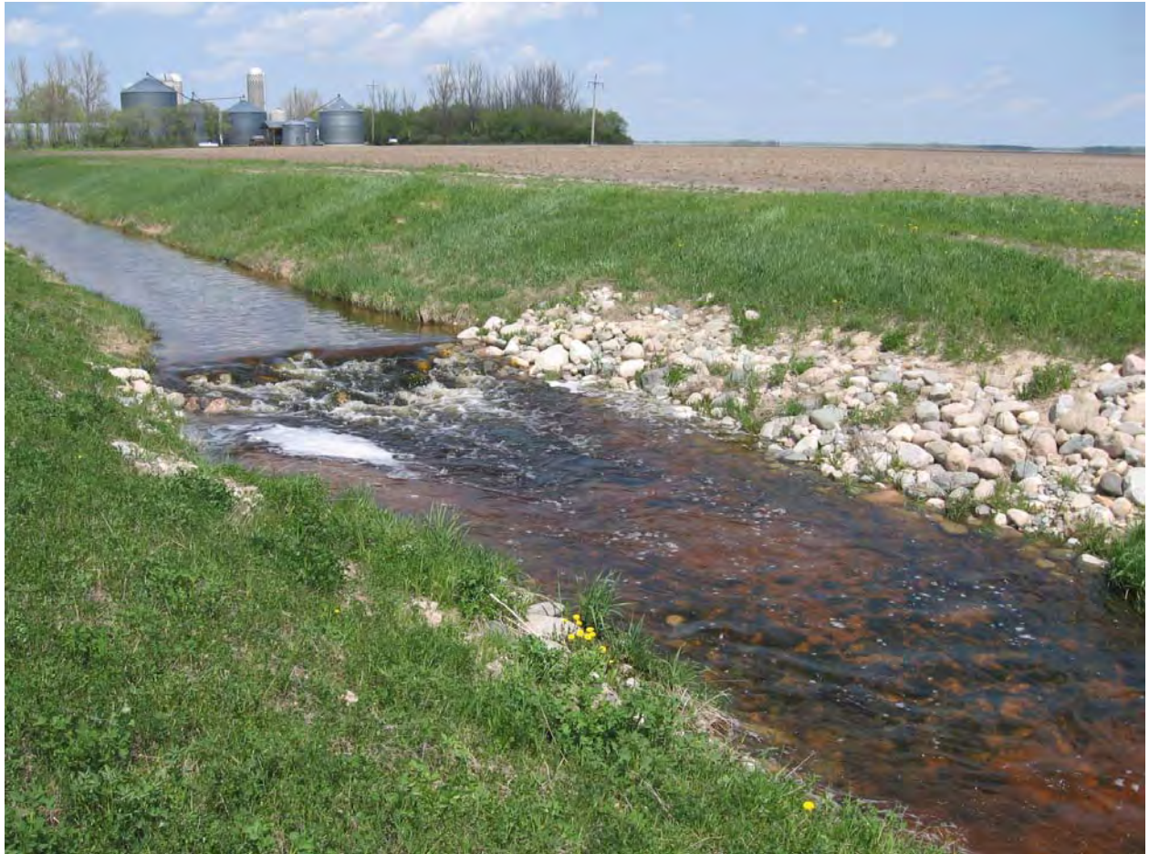
Figure 171. Example of a grade stabilization structure within a ditch.
