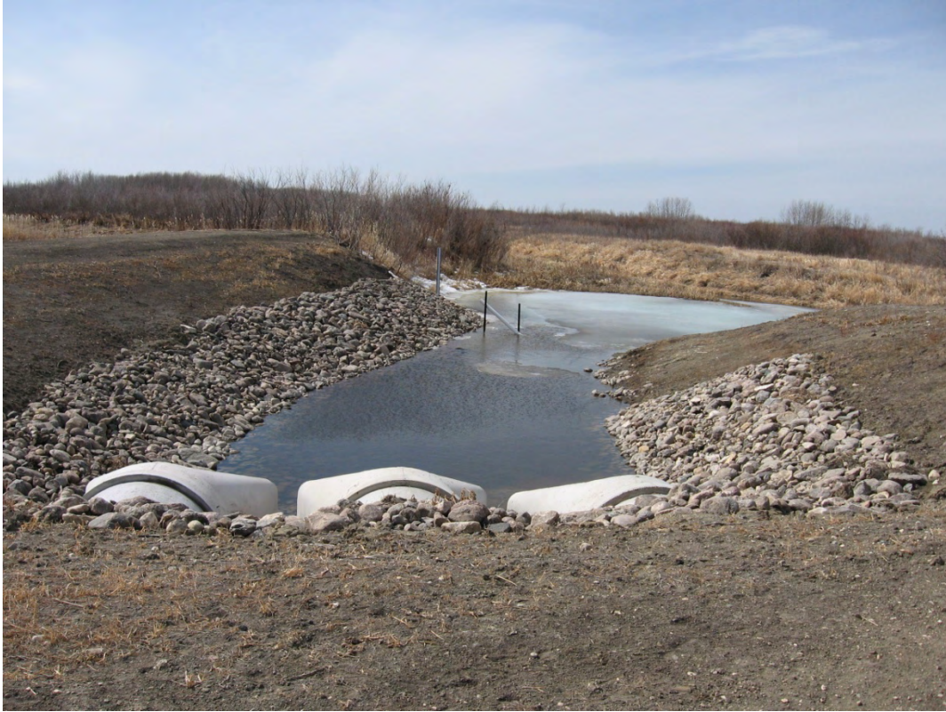
Figure 176. New outlet for Agassiz Pool (Site A5)
