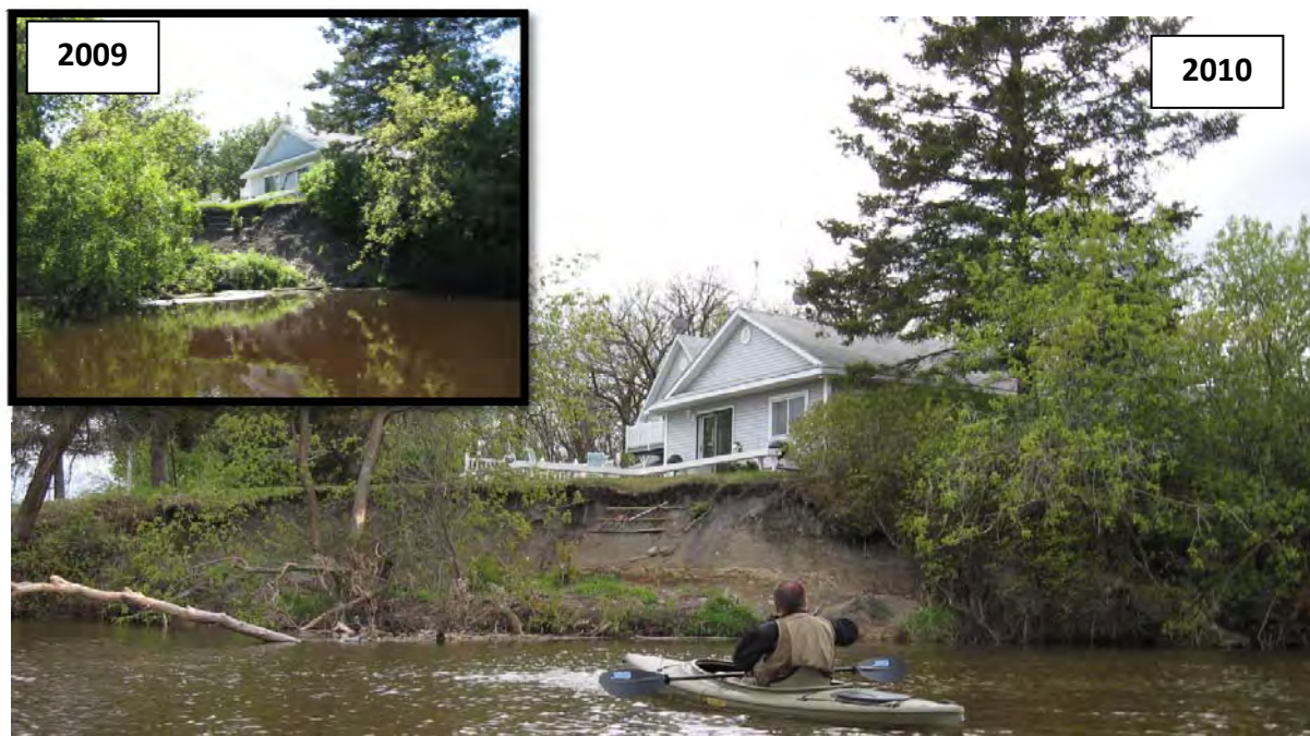
Figure 175. Actively eroding cutbank nearing a home.
