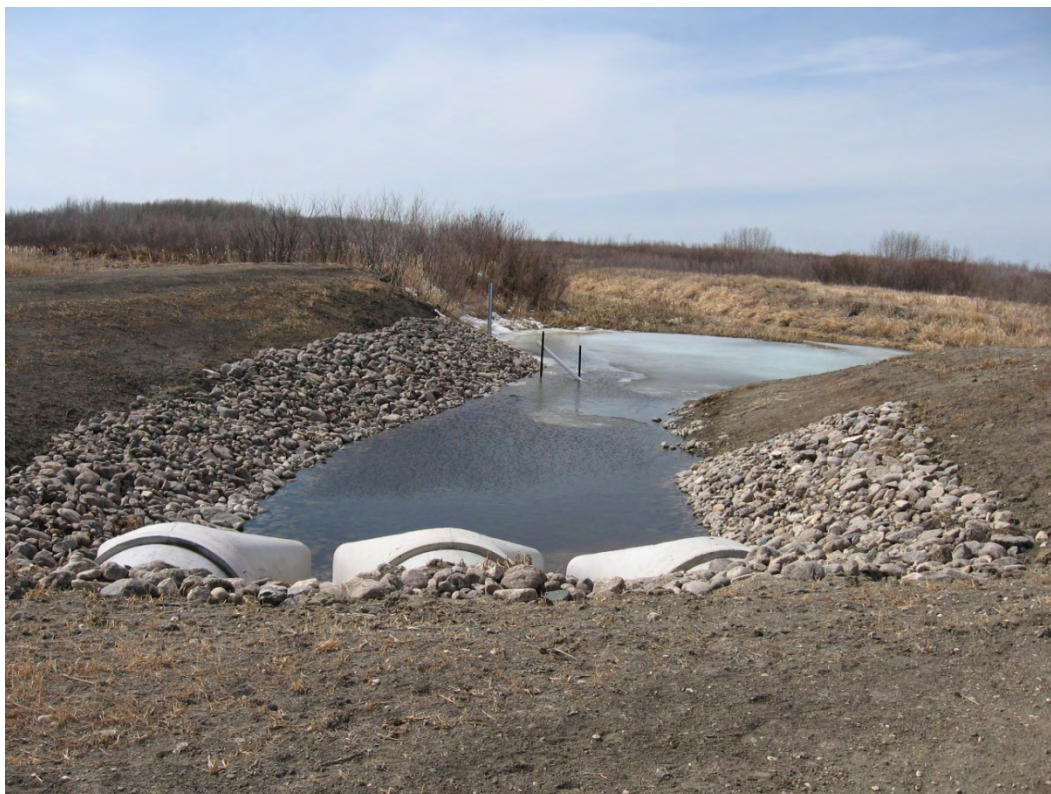
Figure 13. A5 outlet (new Thief River/SD83 outlet structure).
